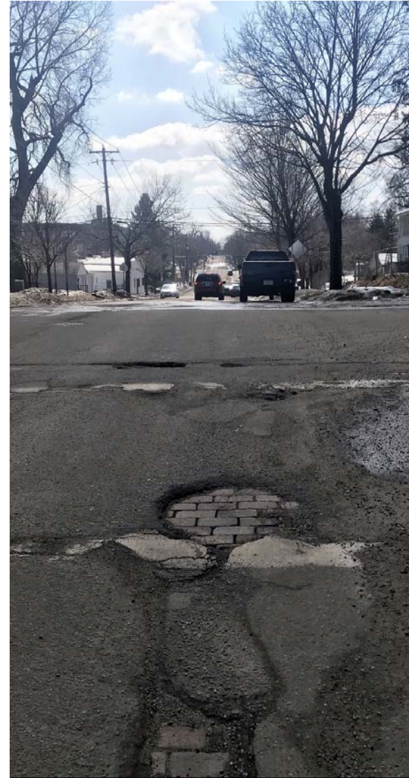
Along Earl Street
