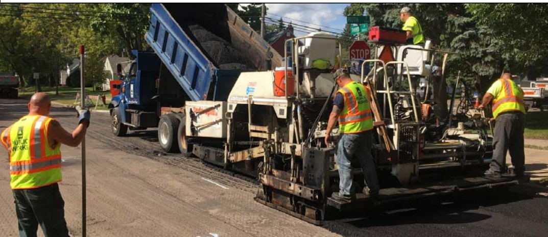
Mill and Overlay
