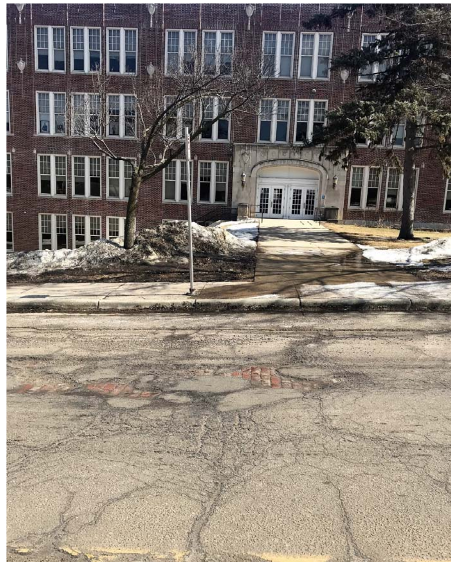
Along Earl Street near 3 rd Street East
