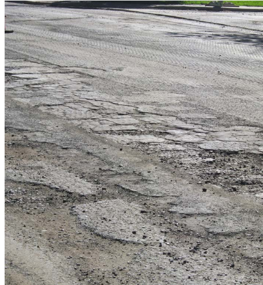
Fairview Avenue near Highland Parkway in 2010 after the roadway was milled. Current PCI is 47 just 9 years after this mill/overlay occurred.
