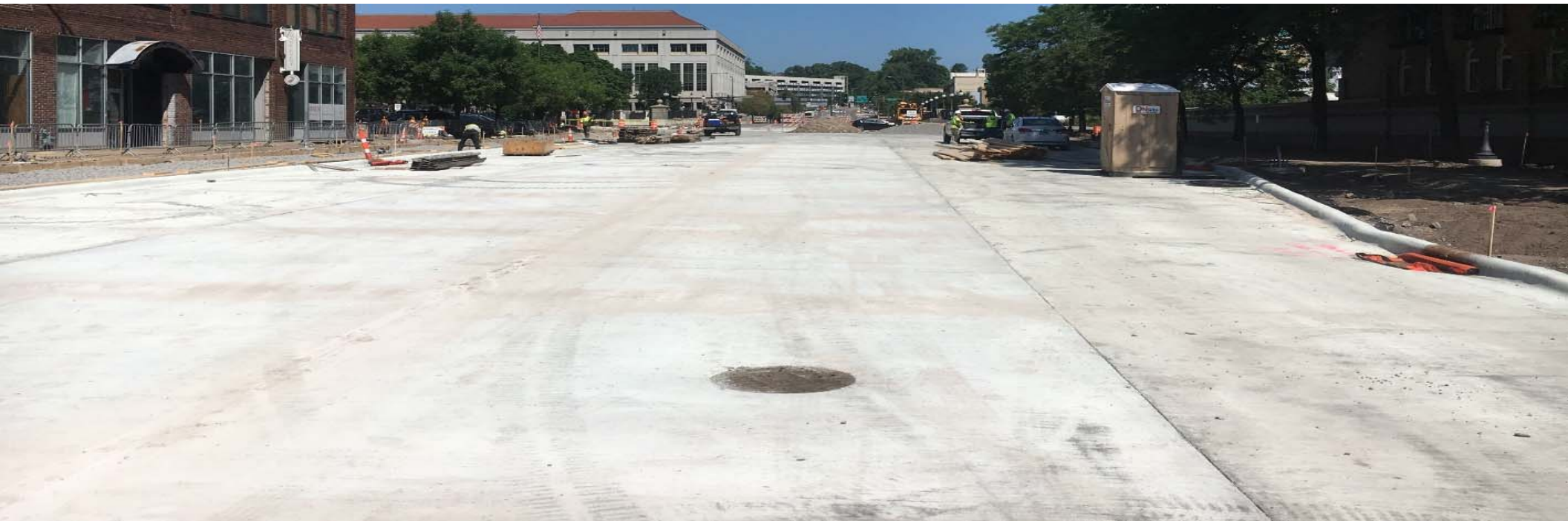
The Jackson Street Reconstruction Project
