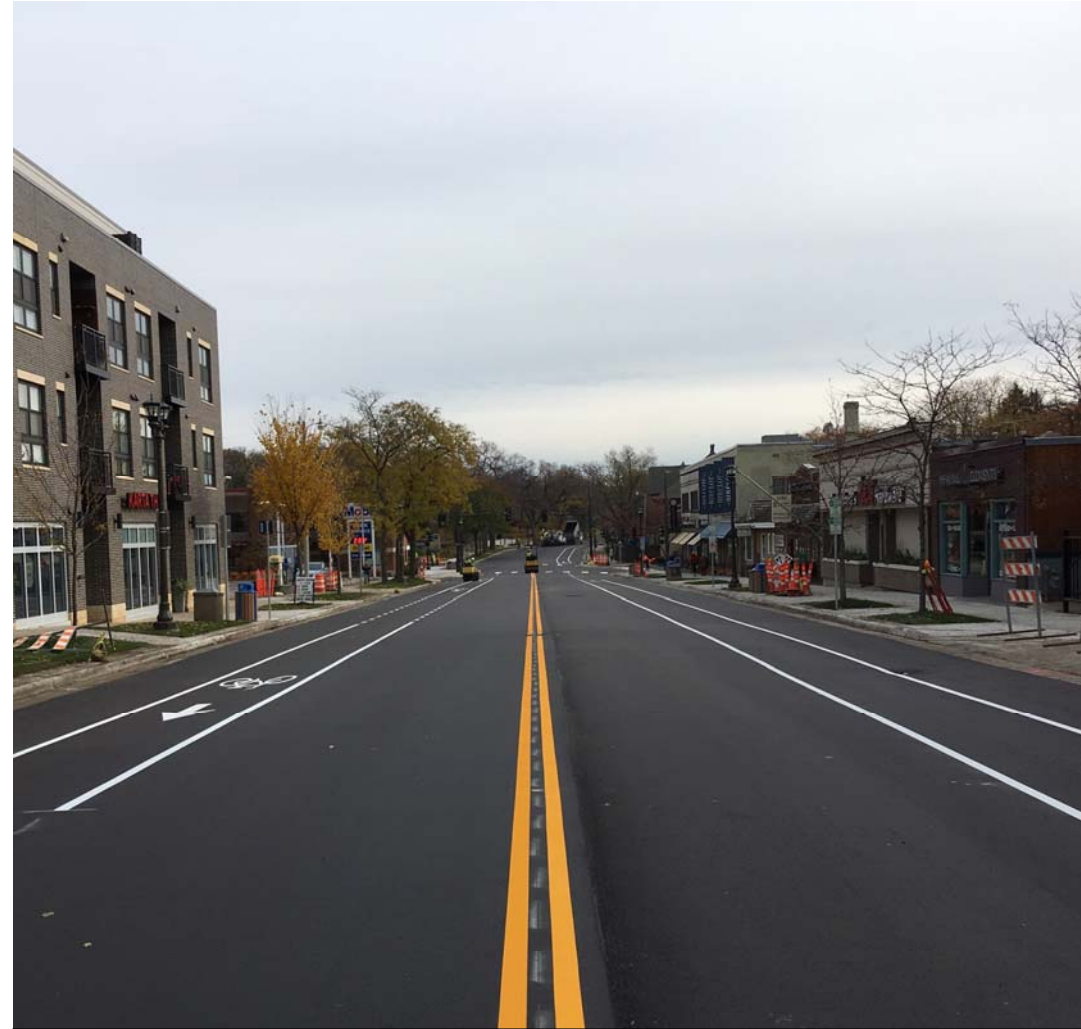
Newly constructed Como Avenue is a good example of how a reconstruction project can help improve the non-motorized environment.
