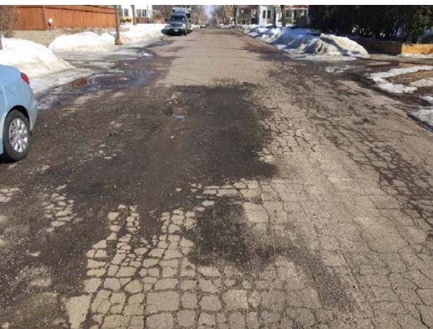
PCI = 40 (Poor)
